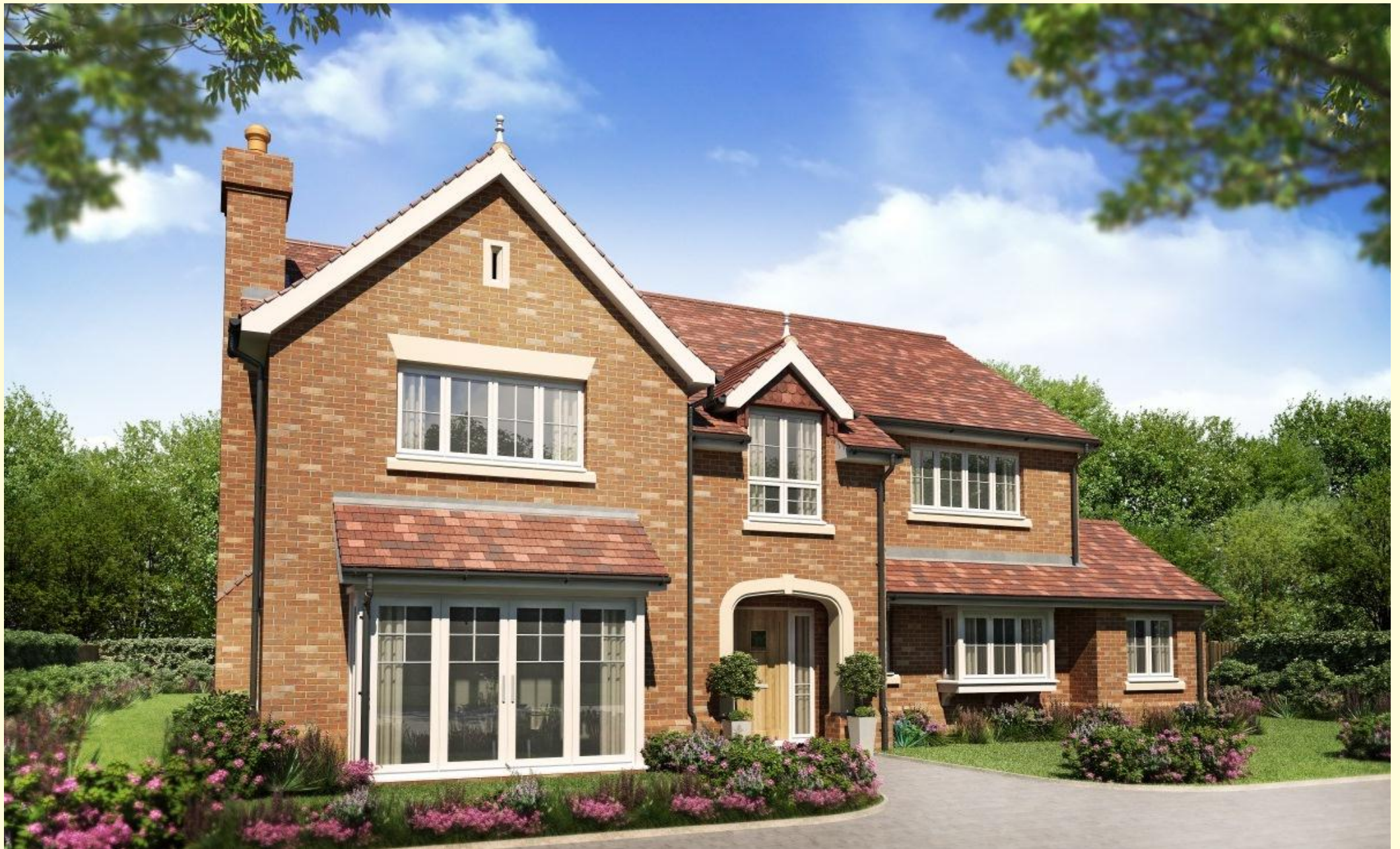
Highgrove House, Drews Park, Beaconsfield
